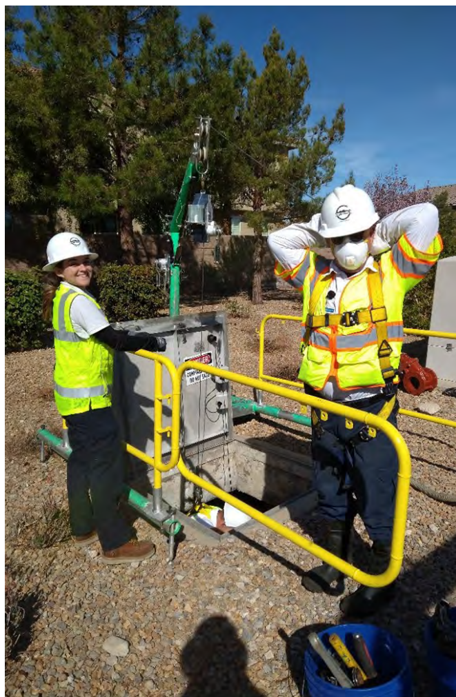
Staff replacing an underground meter
