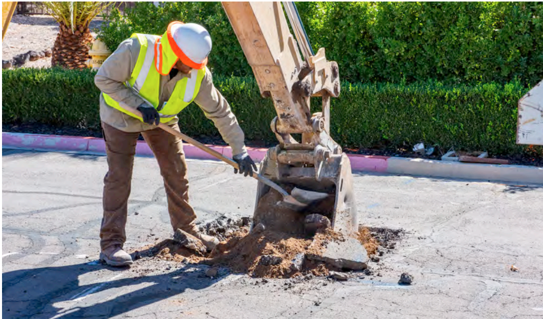
Staff replacing a service lateral
