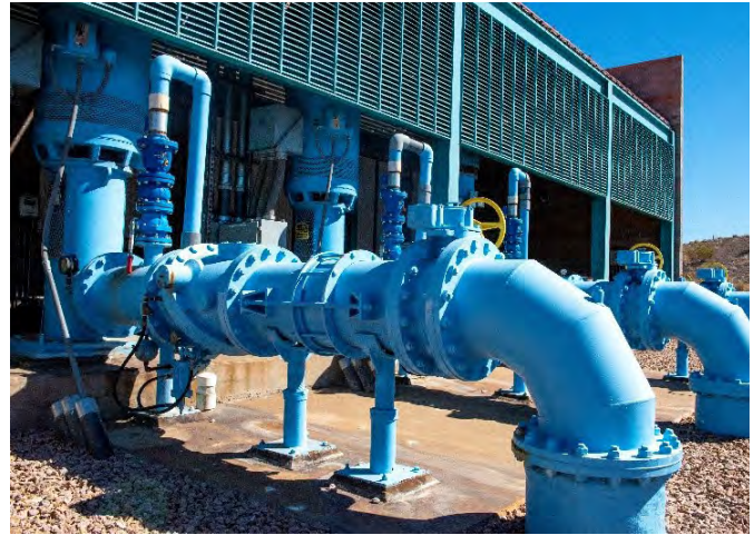
Clearwell pumps at Water Treatment Plant
