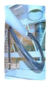
For example, if the flexible piping product allows a maximum of four 90° bends, then the equivalent length must be less than or equal to four 1" 90° elbows, which is 8 ft. (4 x 2 feet per NFPA 13 Table 22.4.3.1.1)
