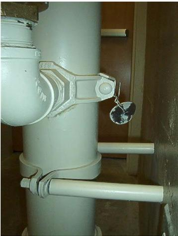
NFPA 13 - 6.5.5.2 (as amended) "When hole cutting or drilling of pipe is done **in the field**, debris discs shall be retrieved and attached to the piping at the point at which the hole was made."
