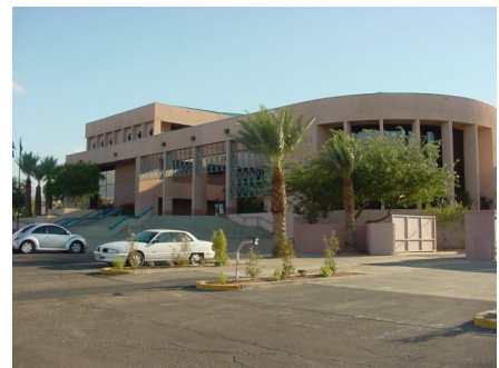
Figure 34—City Hall parking on Water Street.
