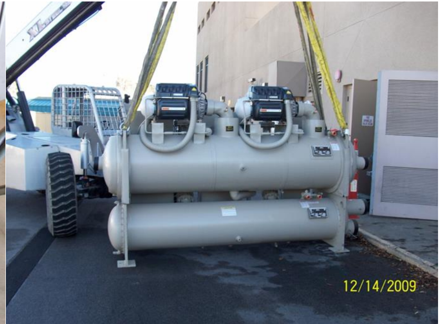
200 Ton Magnetic bearing, Frictionless McQuay Chiller ready for install
