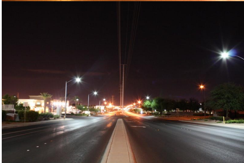
Gibson Road lighting
