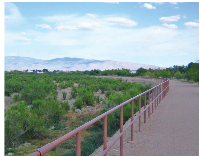
Figure 27 Railings. Railings and guardrails can still meet safety criteria while minimally intruding on the trail experience. Custom railing details at key locations can be tied into the overall theme of the trail system.
