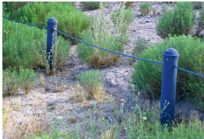
Figure 25 Example barrier fencing. Design uses durable materials, successfully contains users and minimally intrudes visually on the trail experience.
