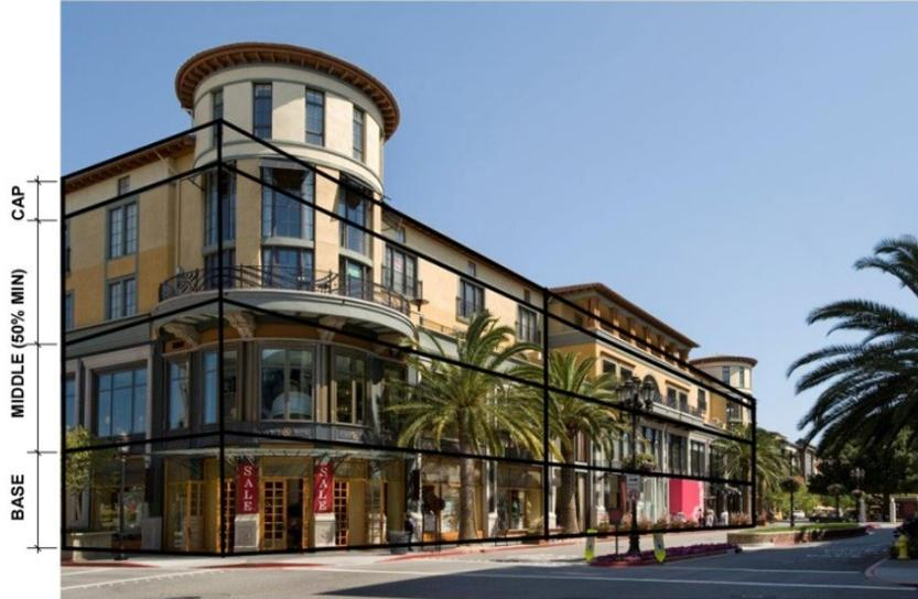
Figure 5.2.1: Example of Base, Middle, and Cap design
